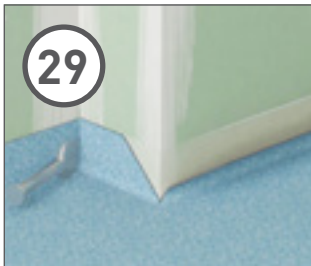
29 Push the flooring edges firmly into the corners.
