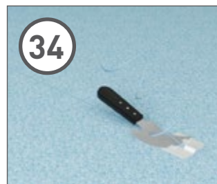
34 Trim the welded joints in two passes using a trim plate or sharp knife.
