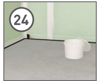
24 Brush pre-mixed reactive adhesive on to the walls.
